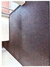
21. Lounge room - Floor/floor coverings 21/05/26 at 10:09 AM
