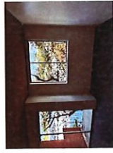
5. Lounge room - Doors/walls/ceiling 21/05/26 at 10:05 AM
