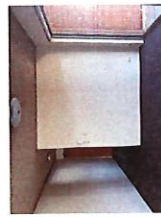
1. Lounge room - Doors/walls/ceiling 21/05/26 at 10:04 AM
