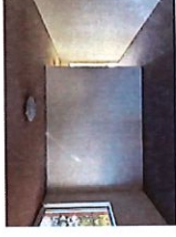
4. Lounge room - Doors/walls/ceiling 21/05/26 at 10:04 AM
