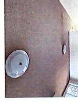
7. Lounge room - Doors/walls/ceiling 21/05/26 at 10:05 AM
