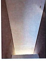
3. Lounge room - Doors/walls/ceiling 21/05/26 at 10:04 AM
